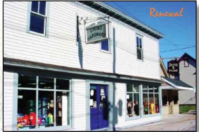
Chums a local hardware store after renewal
